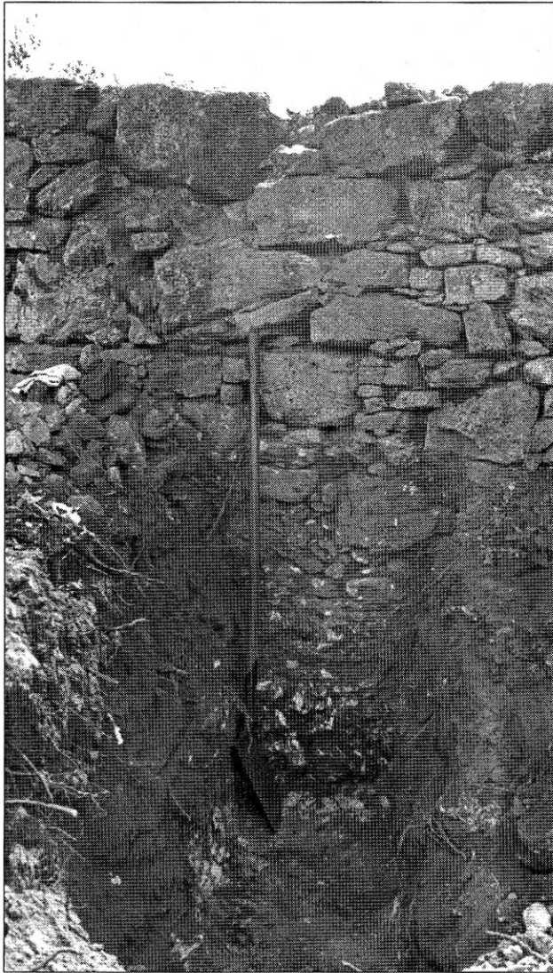
Figure A-47. Trench in midden deposit, showing stone fence 7'2" tall that enclosed Aranama Mission. The deposit at this point is 40 inches deep, with the fence extending 46 inches above. Courtesy TARL, UT-Austin, photo 41GD1-15.
